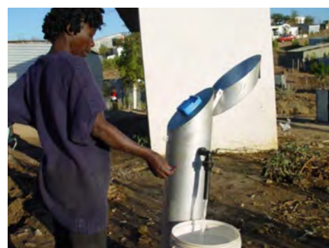
Figure 10.12 Metered and un-metered community standpipe
