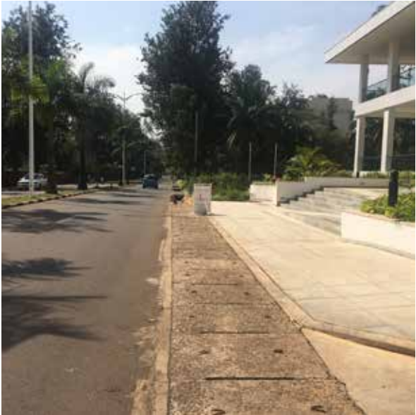
Existing road infrastructure - storm water channel
