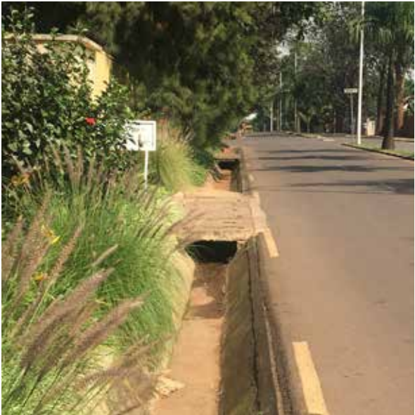
Existing road infratstructure - storm water channel
